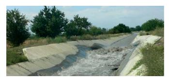
The Khanarc Canal was designed so that water flows under gravity, saving the expense of pumping.
