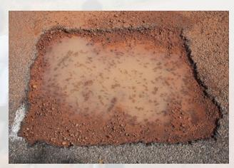
While waiting for maintenance work to start, road authorities cut potholes into rectangular shapes. This temporary measure helps to disperse any water that has collected across a larger area, which reduces the extent to which it deepens the hole.
